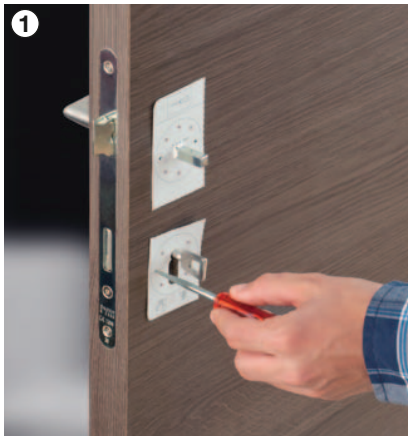
1 Fix the template on the door by inserting the key into the keyhole and mark the bores for the guiding lugs.
