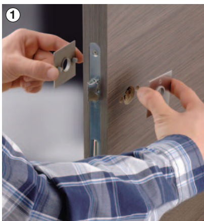
1 Place the handle roses in position
