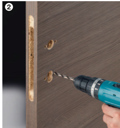
2 Drill the holes for the guiding lugs (remove the lock case for this).
