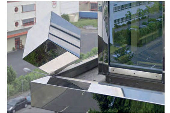
Bright annealed facade cladding before and after cleaning: Standard maintenance operations return the highly reflective surface to its original lustre. Photo: Christian Pohl GmbH, Cologne (D)
